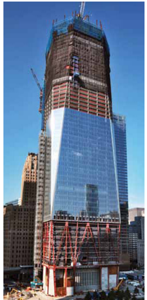
1WTC Construction, June 2011. Courtesy of Joe Woolhead
